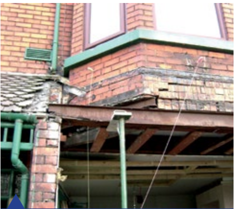
Rotten steel supports
