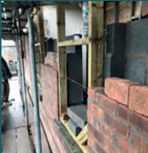
Photo 10: New cavity wall, internal dense block, insulation, wall ties & facing brick
