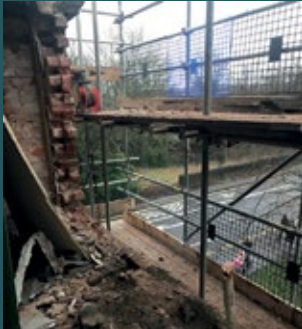
Photo 9: Visible chimney flues & solid 9 inch wall
