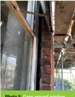
Photo 5: Gaps around window, sill and lintels in gable wall showing 100mm outward bulge.
