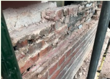
Photo 6: Solid 9" wall with crumbling mortar in poor condition
