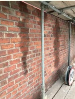
Photo 1: Gable wall cavity holding water
