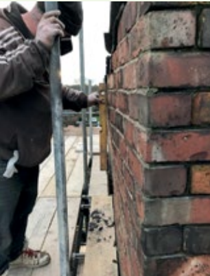
Photo 2: Chimney stack leaning
