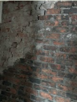
Photo 3: Internal wall cracking
