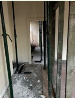
Photo 4: Floor to gable separation along the left side
