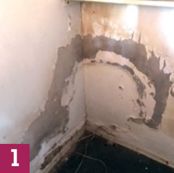
Rising damp sulphide ‘tide mark’
