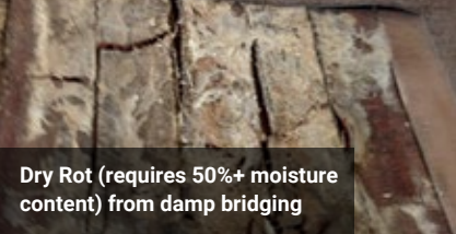
12 Dry Rot (requires 50%+ moisture content) from damp bridging
