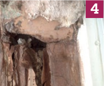
Prolonged plaster/masonry damage from rising damp in empty auction property.
