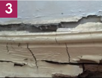
Wet rot (requires 30% moisture content) from rising damp bridging from floor slab with no DPC sheet or insulation.
